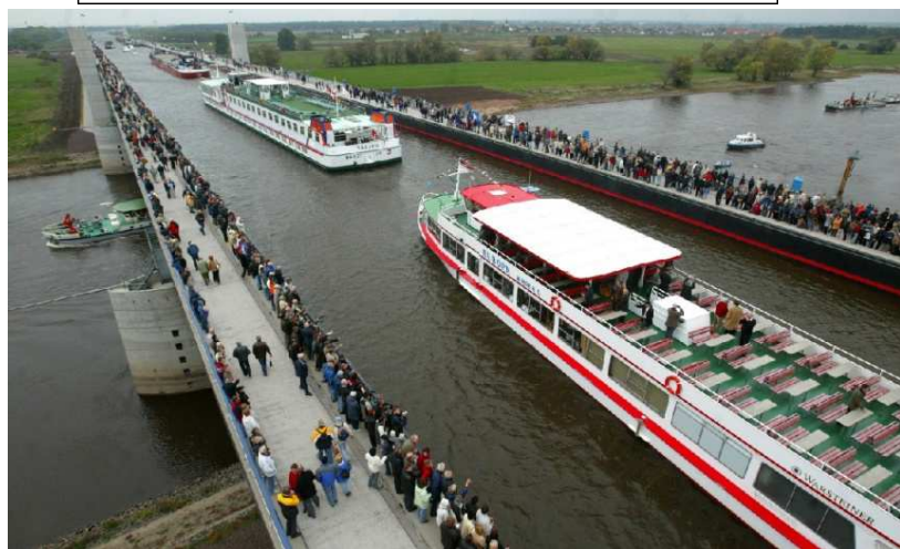
River Crossing – Minden, Elbe, Germany
